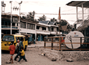
Fig. 1: VSAT Telphony at a Public Internet Service Station
