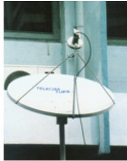
Gambar 3b. One-way satellite Internet access with 1.2 meters antenna receive only
