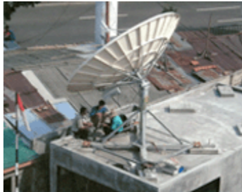
Bangladesh ISP installing VSAT antenna to access USA Internet backbone.
