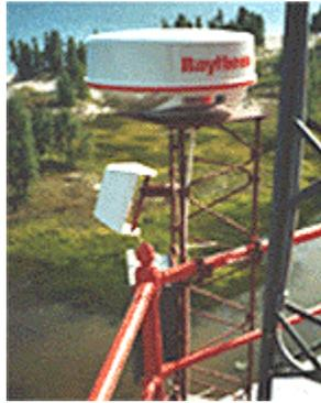
The radar system and the satellite earth station installed on the lighthouse at Longpoint
